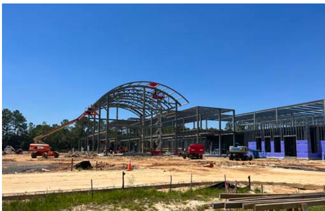
October 2023: The STHS Surgery Center continues to take shape.
