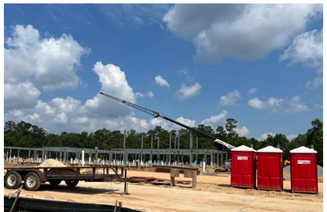
June 2023: Structural steel goes up on the STHS Surgery Center site.
